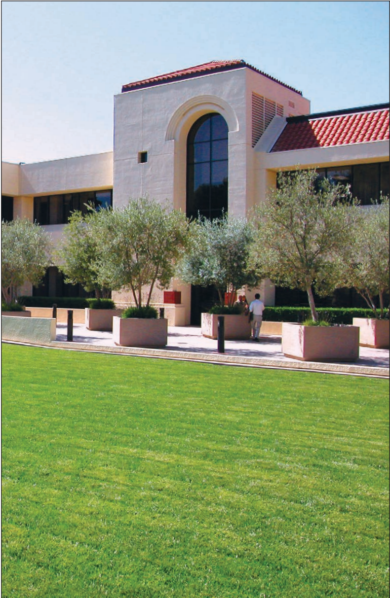
The Caruso School of Law School of Law building is nestled on the hillside in Malibu and is home to the joint Juris Doctor and Master of Dispute Resolution programs.
